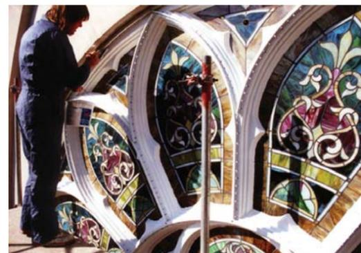
This rose window aluminum protective glazing system was designed to match the frame's tracery in an outset system at First United Methodist Church, Iowa City, IA.
