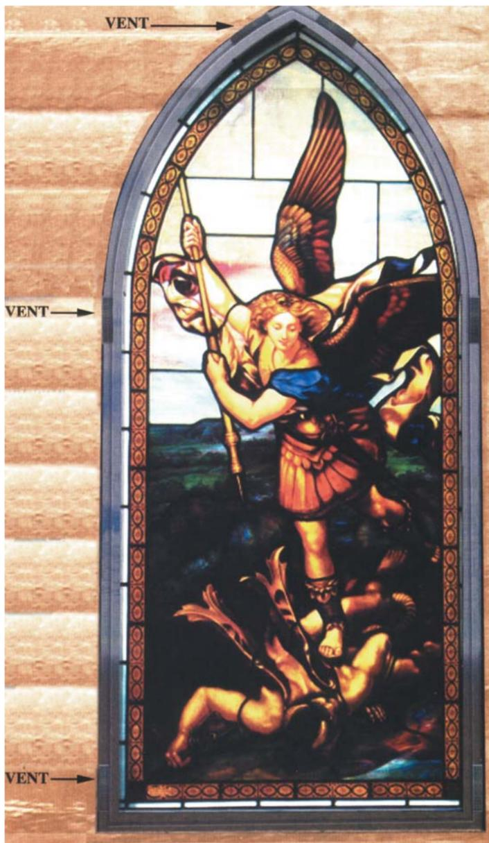
An aluminum-frame ventilation system was installed in this stained-glass window in a private chapel in Wichita, KS.
